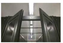
Combining the Cool Pool with the AFPS system guarantees the direct management of the air flow within the cold aisle and optimizing it depending on the variation in load.
